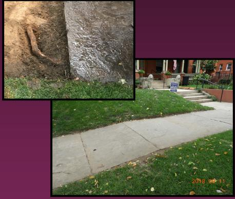
I wanted to cut out the root that was heaving my sidewalk. The Forester convinced me to build a shallow ramp to bridge over the root. This approach eliminated the tripping hazard but still allowed the tree root to thrive.
