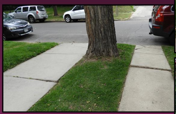
If a portion of the sidewalk is shattered or if it is heaved and offset by more than 3/4", the homeowner must replace or re-level it.
